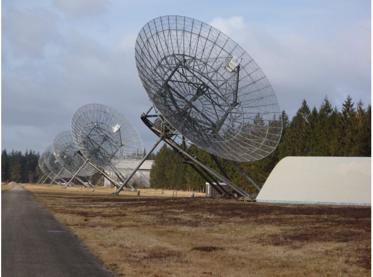
Figure A.3: The Westerbork synthesis radio telescope (WSRT) - the Netherlands. The grey building in the bottom right corner of the picture is the EMBRACE (Electronic MultiBeam Radio Astronomy ConcEpt) dome. EMBRACE is an aperture-plane phased-array prototype using tiles of Vivaldi feed antennas. It is part of the FP6 European Project SKADS [93] and it has installations at Westerbork and Nancay.
