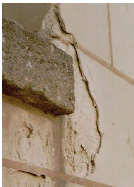
Fig. I-16. Stone degradation by contour scaling, Castle of Chambord, France (tuffeau limestone) (Beck, 2006).
